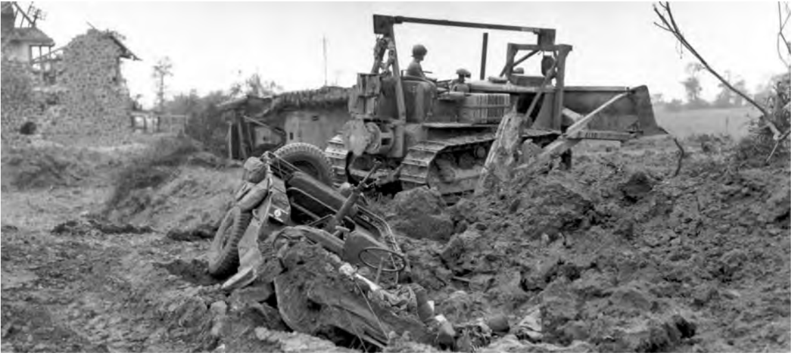
A BULLDOZER (tractor, earth moving crawler, diesel) pulling a jeep from a crater (top). Engineers using a truck-mounted revolving crane swing a section of a tread-way bridge into place over the Vire River near Pontfarcy (bottom).
