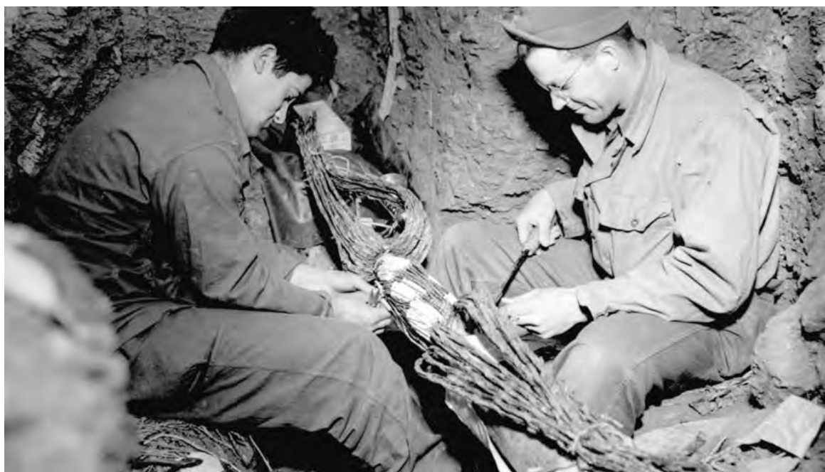
TWO TYPES OF MINE DETECTORS. At left, AN/PRS-1 type; at right, SCR 625 (top). Mine detectors were developed by the Signal Corps primarily for use by Engineer troops. Signal Corps repairmen splicing wires of an underground cable which was damaged by artillery fire (bottom).
