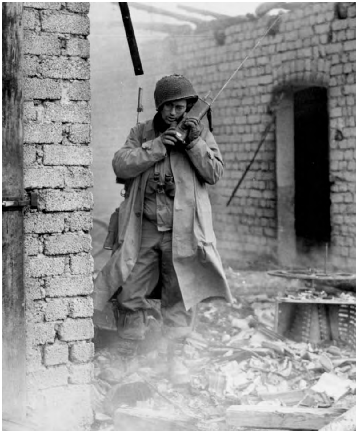
HANDIE-TALKIE. An infantryman, armed with a carbine equipped with a grenade launcher M8, using a handie-talkie radio SCR 536.
