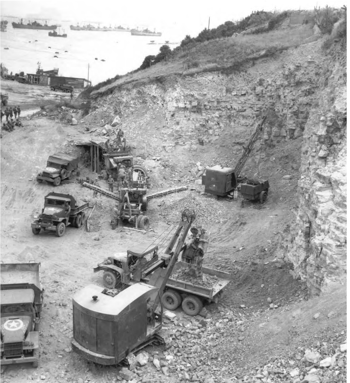
A QUARRY NEAR OMAHA BEACH used by engineer units to supply rock and stone for the construction of roads. The tremendous amount of traffic on the roads in Normandy, as men and supplies were brought into France over the beaches required the services of many engineer units to keep the roads in good repair. Most of the roads leading to the beaches were not hard surfaced but were constructed of rock and gravel.
