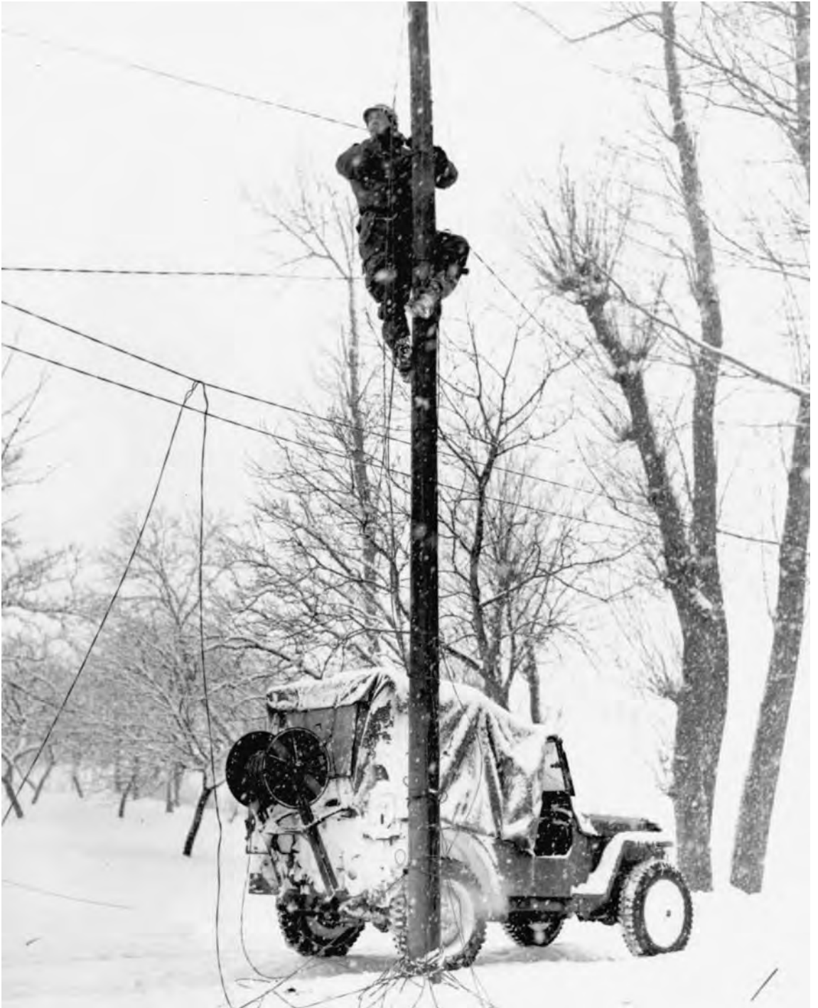
A SIGNAL CORPS LINEMAN repairing damaged telephone lines.
