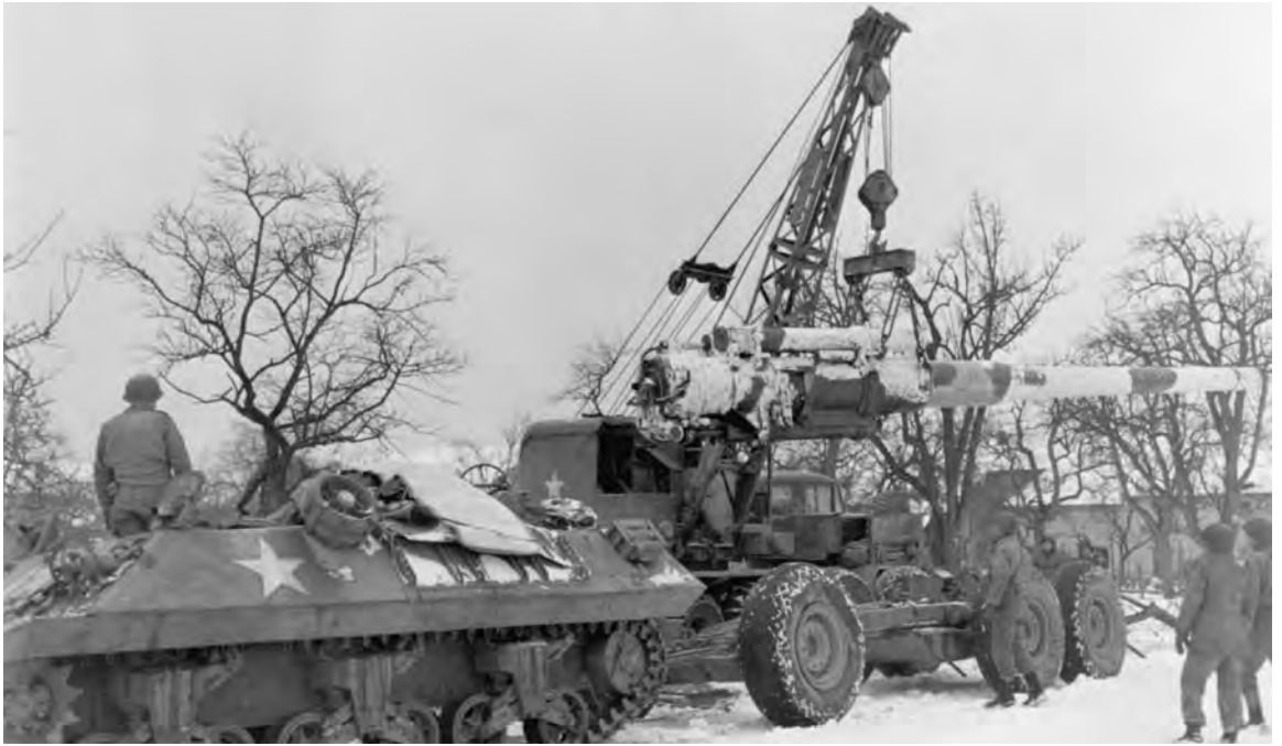
A TRUCK-MOUNTED CRANE swinging the barrel of an 8-inch gun from its transport wagon (top), and placing it on its carriage (bottom). The gun and cradle were transported on one vehicle and the carriage on another.
