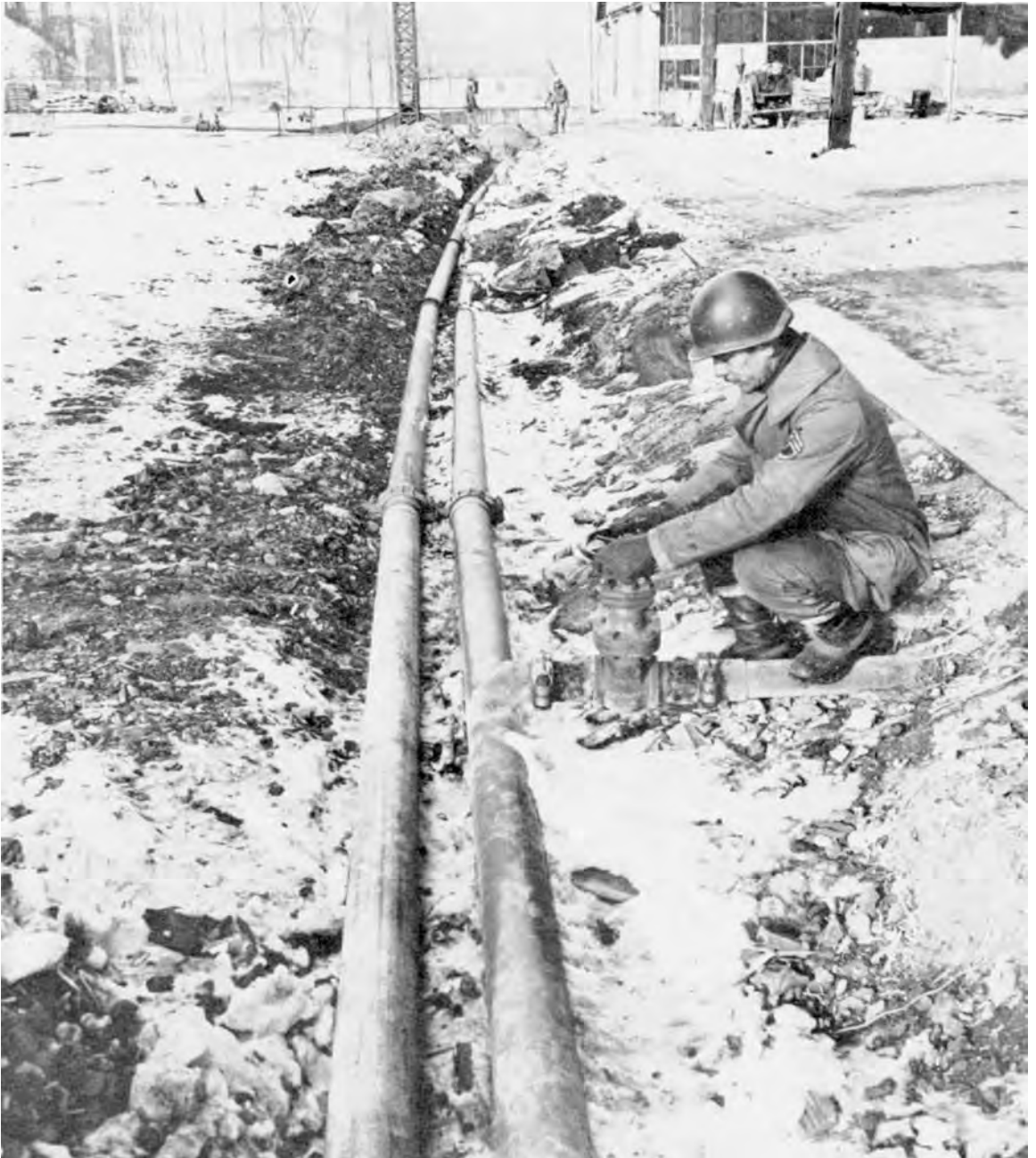
OPENING THE VALVE ON A GASOLINE PIPELINE. The critical fuel situation of September, which had stalled the armored divisions at the West Wall, was materially improved by December. At that time three main pipelines were constructed or under construction: one for the northern armies, one for the central armies, and another for the southern armies.
