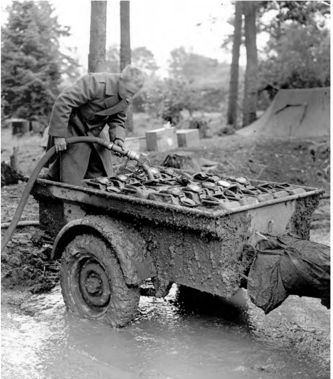
FIVE-GALLON WATER CANS loaded in a quarter-ton trailer being filled at an Engineer water point. The Engineers were responsible for the purification of drinking water and set up water points from which all units located in the area drew their daily supply.
