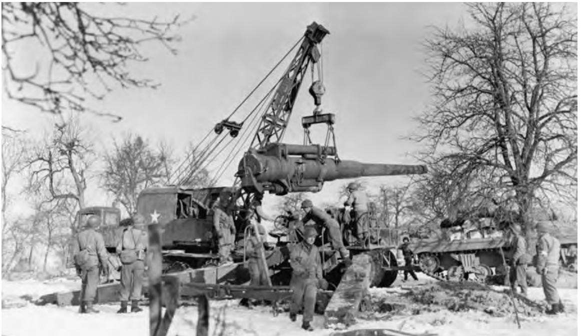
A TRUCK-MOUNTED CRANE swinging the barrel of an 8-inch gun from its transport wagon (top), and placing it on its carriage (bottom). The gun and cradle were transported on one vehicle and the carriage on another.
