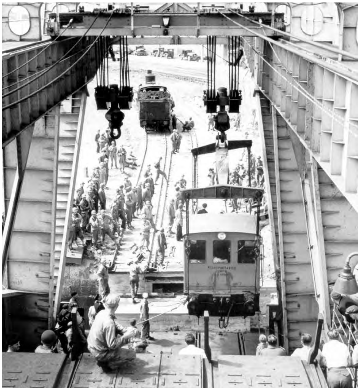
RAILROAD EQUIPMENT BEING UNLOADED FROM A SEATRAN at Cherbourg. Motor convoys could not handle the vast quantities of supplies needed to maintain the Allied fighting forces and it was necessary to supplement these convoys with rail transportation. The first scheduled run was made between Cherbourg and Carentan on 11 July 1944, using mostly salvaged French equipment. As soon as the Cherbourg port facilities were sufficiently restored, equipment was brought over from England and put into service.
