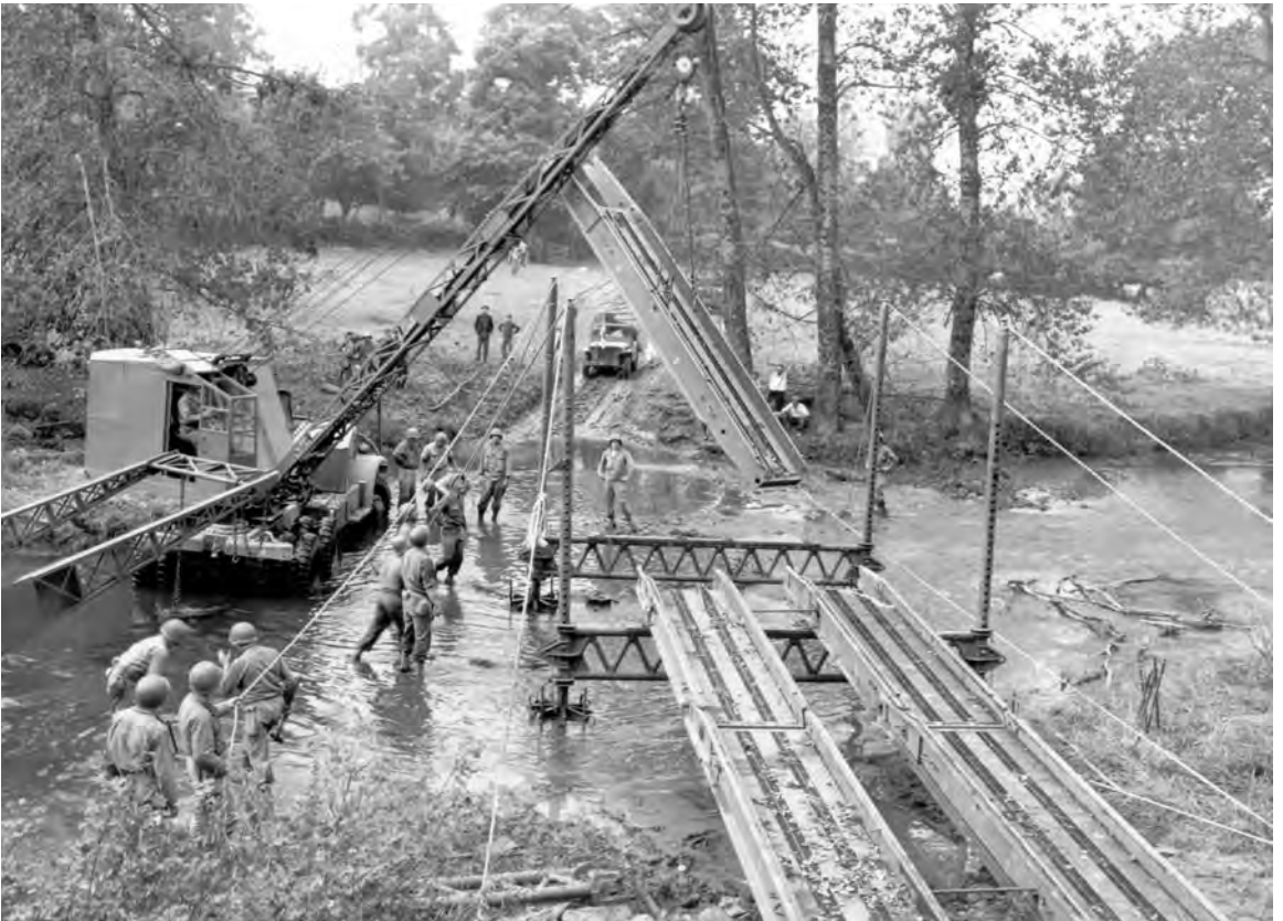
A BULLDOZER (tractor, earth moving crawler, diesel) pulling a jeep from a crater (top). Engineers using a truck-mounted revolving crane swing a section of a tread-way bridge into place over the Vire River near Pontfarcy (bottom).
