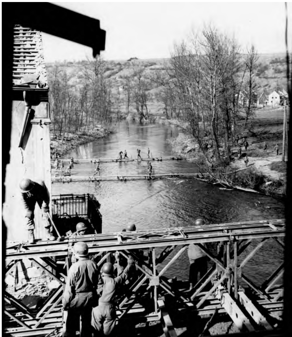
INFANTRYMEN USING FOOTBRIDGES to cross a river while engineers complete a Bailey bridge. On 15 March three corps of the Seventh Army began attacks, one in the heart of the important Saar industrial area around Saarbruecken, the second driving toward Zweibruecken and Bitche, and the third from the Moder River.
